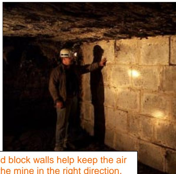
Mine curtains and block walls help keep the air flowing through the mine in the right direction.
