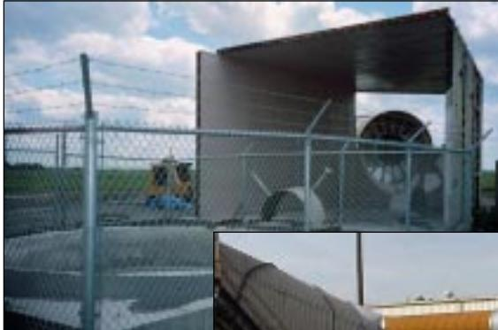
Large fans inside these structures pull air through the mine.
